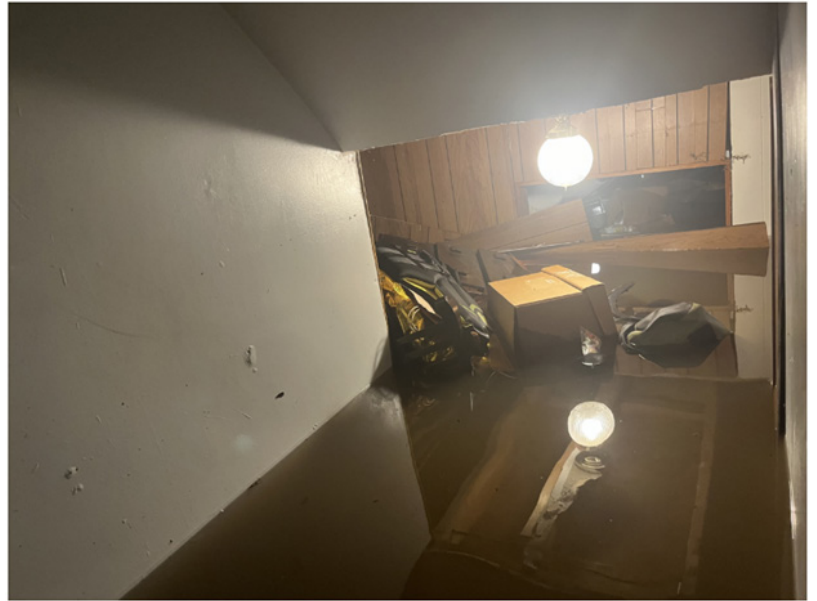
Elizabeth Pelozo's basement following flooding in London, Ontario. Photo submitted
