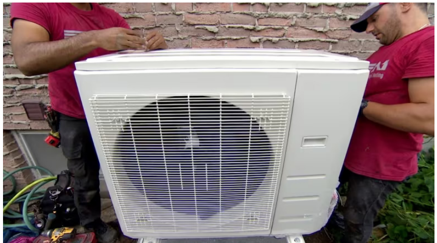
A new pump is installed at a home to replace both an old air conditioner and a natural gas furnace. (Spencer Gallichan-Lowe/CBC)
